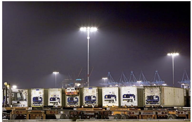
Port of LA; San Pedro, California High Mast System boosted both vertical and horizontal illumination and uniformity that enables a safe working environment.
