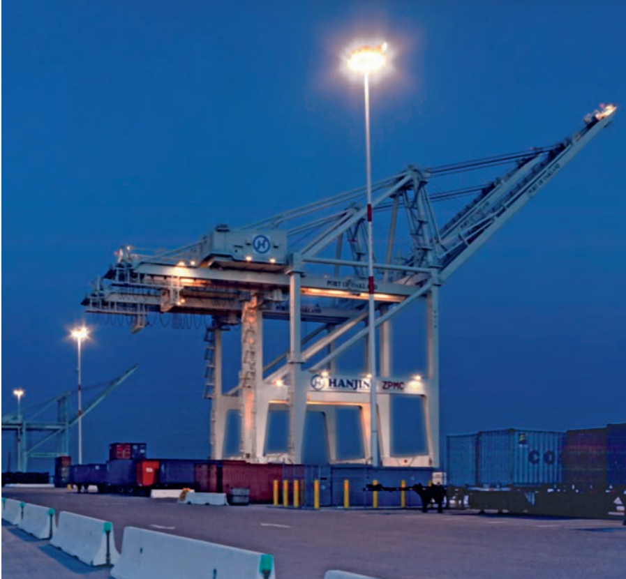
Port of Oakland; Oakland, California The High Mast luminaires have an external shield to eliminate light trespass and meet all Illuminating Engineering Society (IES) full cutoff requirements and the port instituted a restricted uplight policy.
