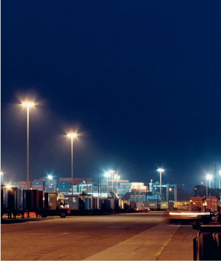
Union Pacific Railroad used two High Mast Systems with 12 luminaires per pole to replace up to 30 wooden poles, which significantly reduced maintenance costs and virtually eliminated downtime. High Mast Systems were used for general lighting, HMSC® luminaires with cutoff optics for areas where light trespass was a concern.
