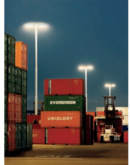
Port of Oakland; Oakland, California The High Mast luminaires have an external shield to eliminate light trespass and meet all Illuminating Engineering Society (IES) full cutoff requirements and the port instituted a restricted uplight policy.
