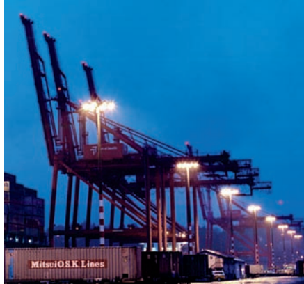
Southwest Harbor, Seattle, Washington The High Mast System has a symmetric and asymmetric distribution to minimize light trespass and glare into the neighboring community without sacrificing visibility which is of particular importance to longshoremen while moving containers.
